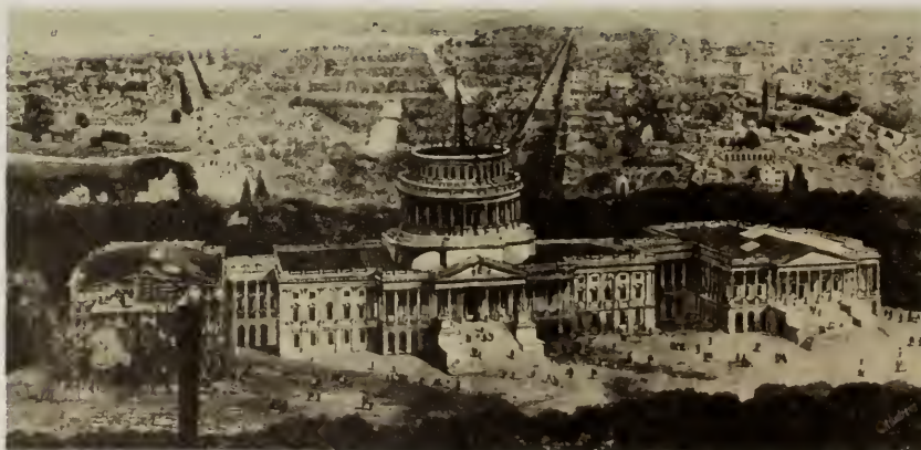
New Senate wing nearly completed, the House wing and the dome still under construction. In May 1861 the Illustrated London News carried this woodcut. It was slightly in advance of the actual progress as the Senate steps and portico had not progressed this far. Tiber Creek runs down the mall toward the half-completed Washington Monument.
